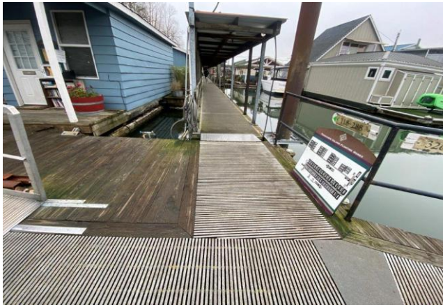
Landing-Top Boards-Wood-Replace
