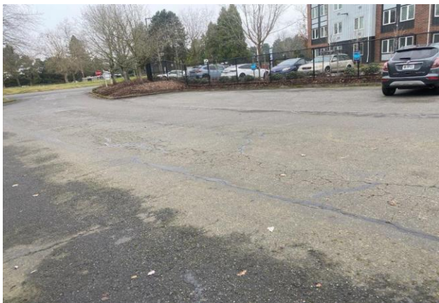
Paving-Asphalt-Repair, Crackseal, Sealcoat
