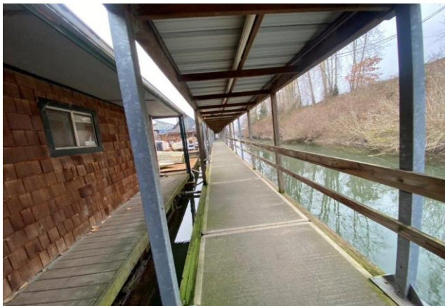
Dock-East-Concrete Safety Repair
