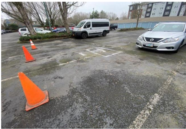
Catch Basin/Parking Lot Drain-Cleanout
